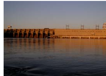
Ice Harbor Dam (photo by Colin Stryker)
